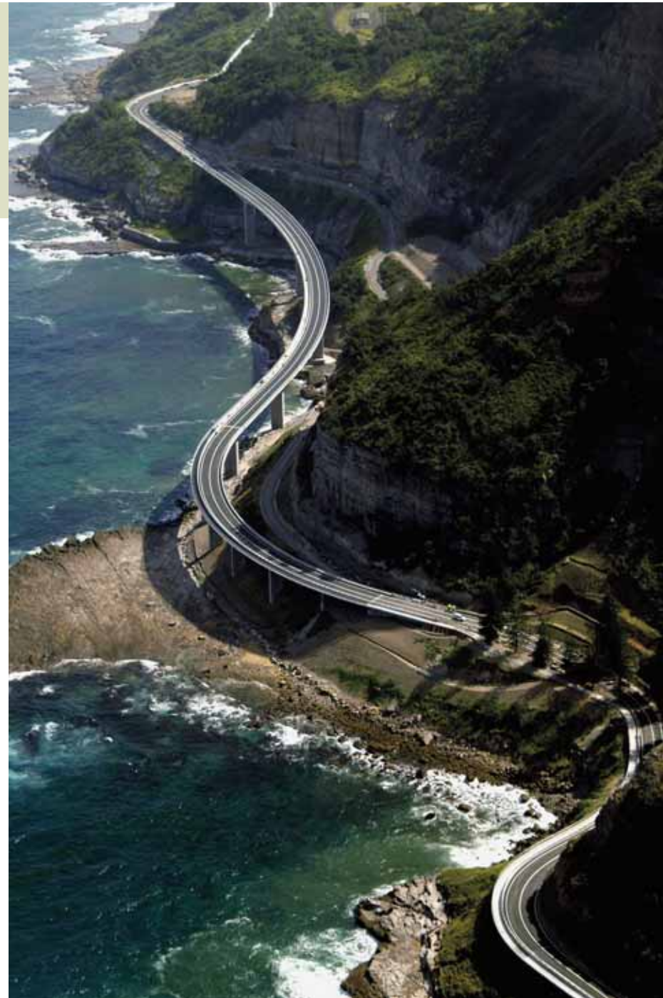
Sea Cliff Bridge, NSW
